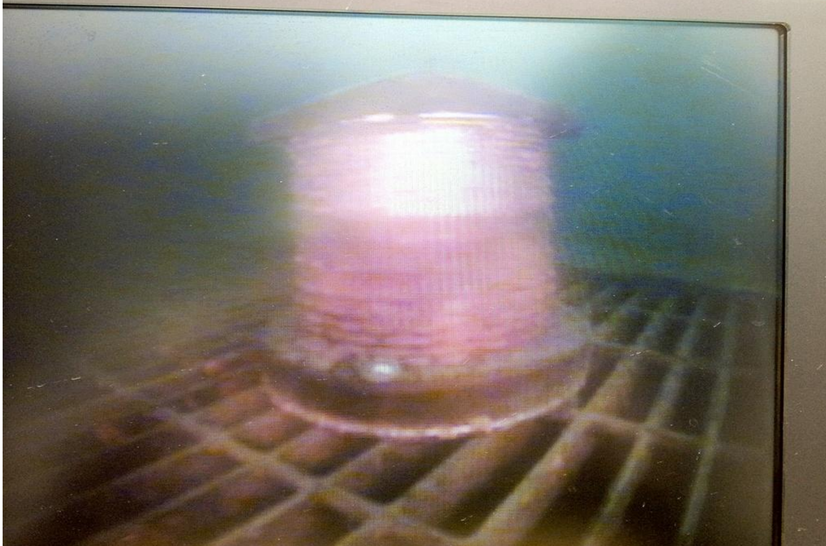
Solar lamp found atop north fishway grating during ROV inspection. Origin unknown. High quality since it was still working.
